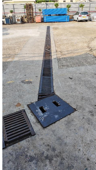
Photo 14: Existing 600 U/C Condition
