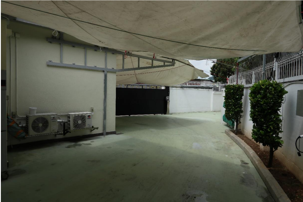
Photographs 23 – Ancillary staff quarters
