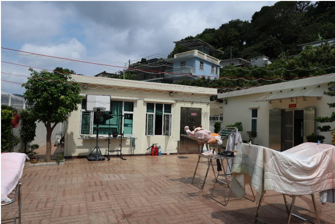
Photographs 22 – Ancillary staff quarters
